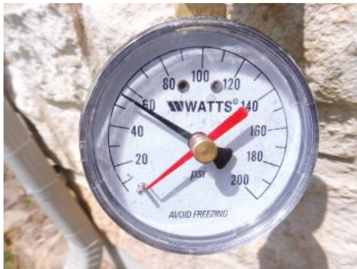
Water pressure was observed to be 55 PSI at time of inspection.
